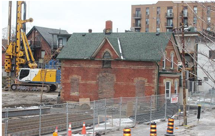
Preparing to move 292 Main Street, December 2020
