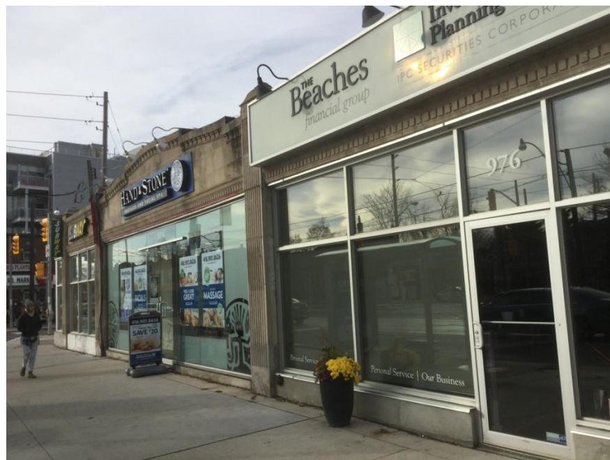
Figure 17. Kingston Road frontage, November 20, 2018.
