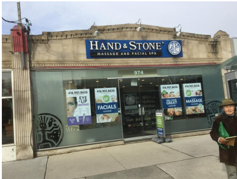
Figure 19. Kingston Road frontage, showing number 974, November 20, 2018. Note that almost all of the red paint from the old Crayons store has been removed (see Figure 21). Photo: Barbara Myrvold
