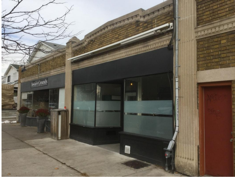
Figure 18. Scarborough Road frontage, November 20, 2018. Note the yellow brick construction in the Flemish bond pattern, the fluted pilasters with conical caps and the two rows of dentils Photo: Barbara Myrvold
